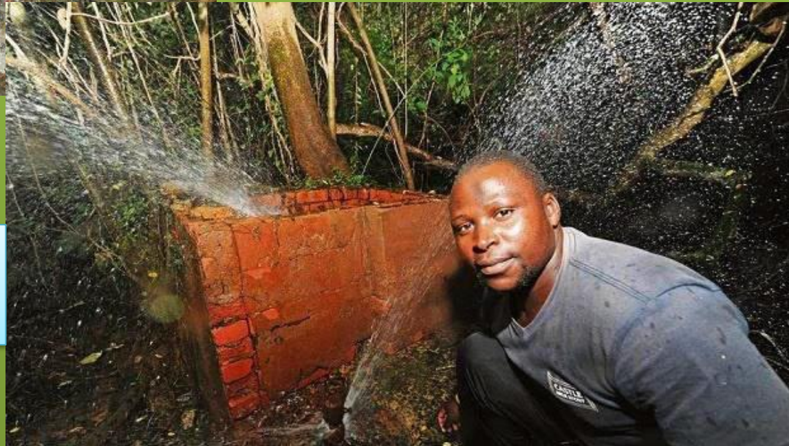
Clean drinking water leakages
